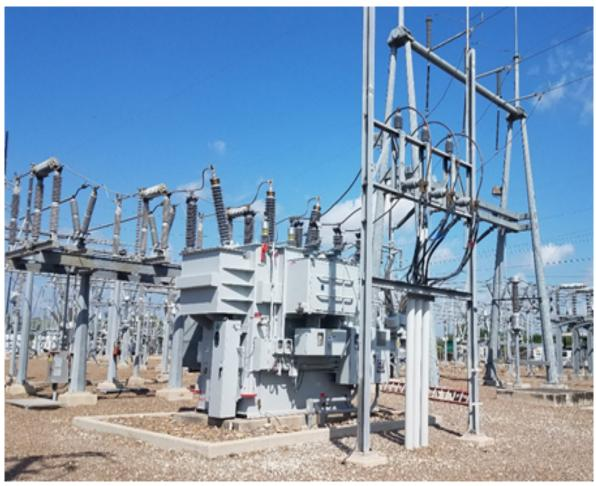
TYPICAL 13.8kv TO 34.5kv TRANSFORMING SUBSTATION
